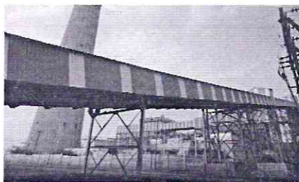
Closed type coal conveying system
